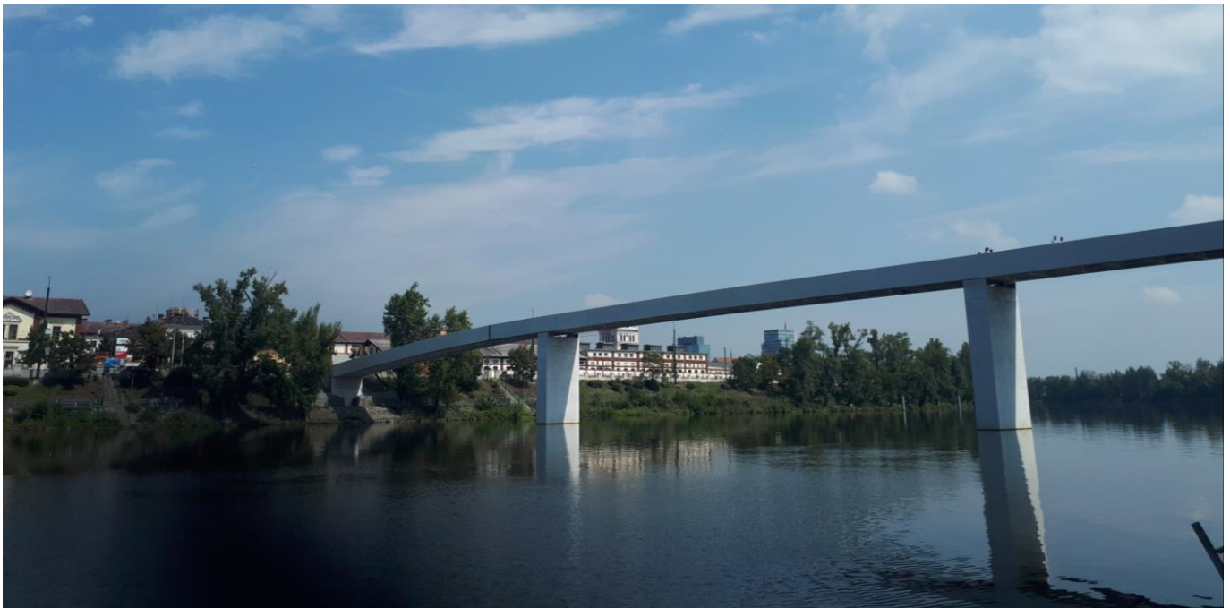
Tuned Mass Dampers on the Stvanice Footbridge over the Vltava River in Prague.
