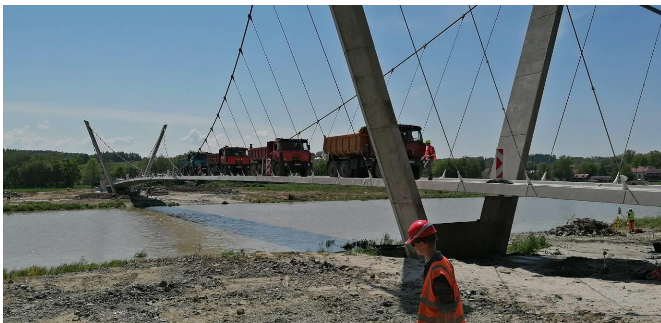
Load test on the footbridge over the River Bečva near Hranice na Moravě, vibration damping by KGF hydraulika (Tuned Mass Dampers – TMDs, vibration absorbers).
