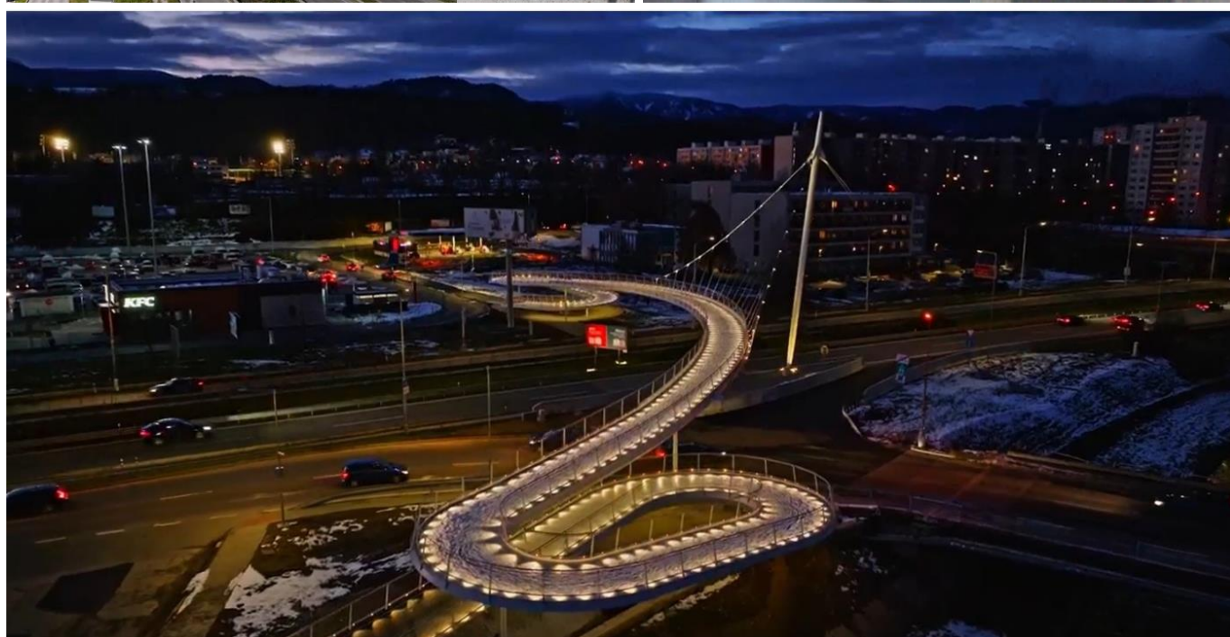
Fluid Viscous Dampers on the Bicycle Bridge over the Elbe River in Celakovice, Czech Republic.
